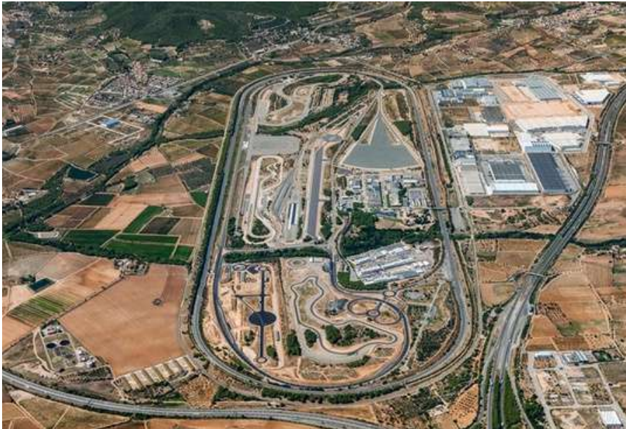
Headquarters & Main Technical Centre
